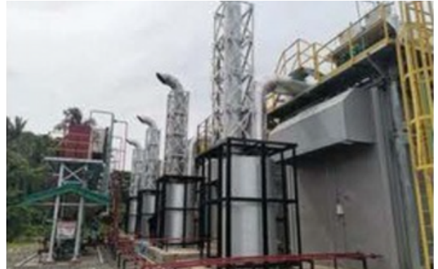
NPC BOAC Diesel Power Plant, Marinduque, Phillipines, 4 x 1.0 MW 8DK-20 Modular Daihatsu Generator
