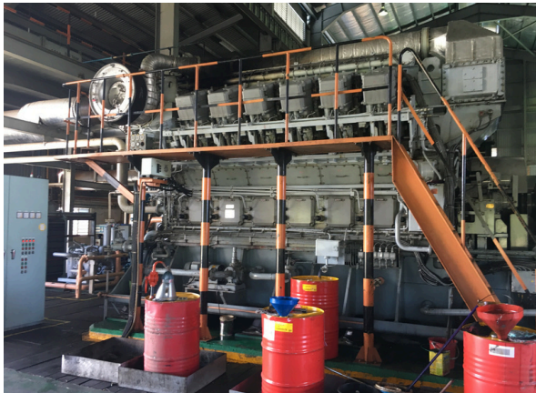
SESCO Limbang New Power Station, Malaysia, Daihatsu Generator 12DK-32B
