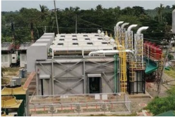
NPC BOAC Diesel Power Plant, Marinduque, Phillipines, 4 x 1.0 MW 8DK-20 Modular Daihatsu Generator
