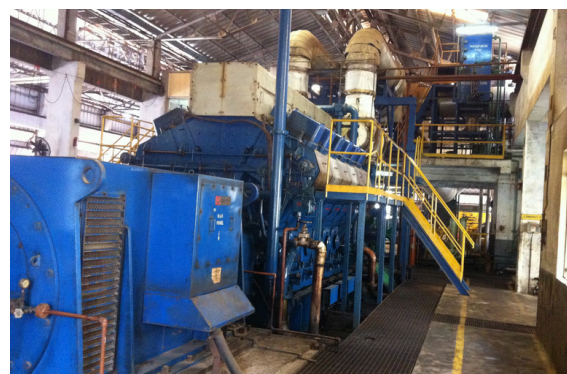
Tube Products of India, Daihatsu Generator 12DK-36
